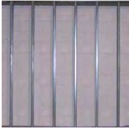
Step 1: Steel Studs
