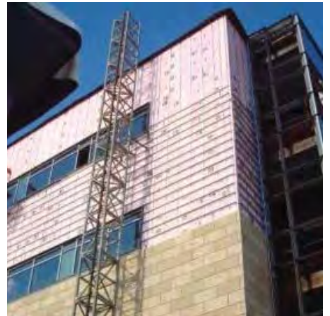
Step 6: Clip Stone on to the Gridworx Channels
