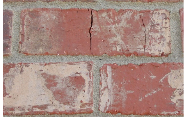
Manufacturing Crack
