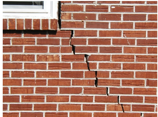
Movement Crack
