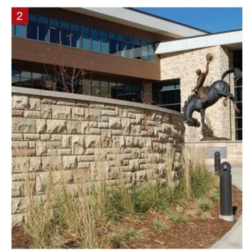
1. Stone installed in a vertical quarter bond pattern | 2. Blend of standard colors (Suede, Café, Garnet) installed in an ashlar pattern.
