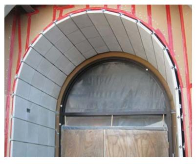
ARRIS•clip, ARRIS•tile and ARRIS•stack do not require a ledge to support the stone veneer units. Overall, these systems are thinner and lighter than traditional brick or stone masonry veneer. ARRIS•clip can also be installed during the winter months without the need for tarps, salamanders and in some cases scaffolding.
