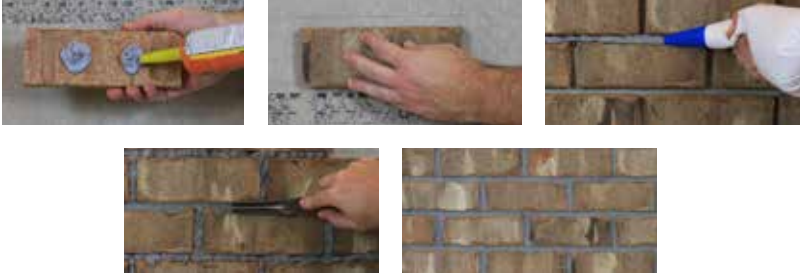
Interior Adhesive Installation
