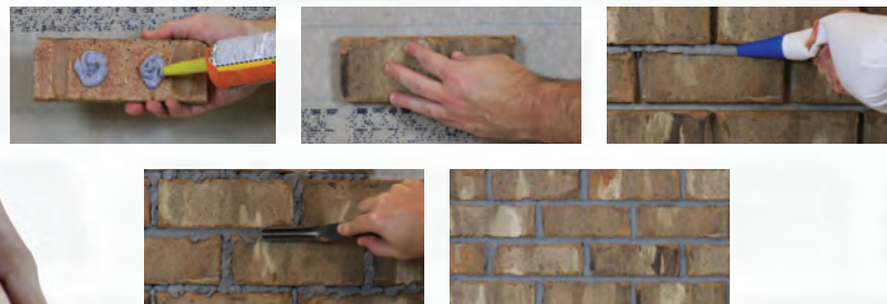
Interior Adhesive Installation
