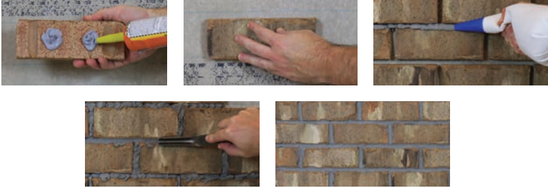
Interior Adhesive Installation
