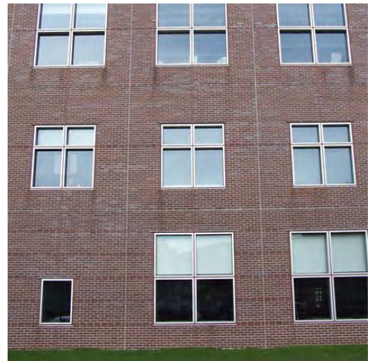
Figure 11: Placement of movement joints creates wall symmetry.
