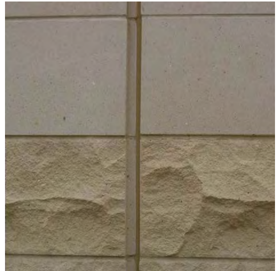
Figure 9: Movement joint placed at continuous notch in veneer.
