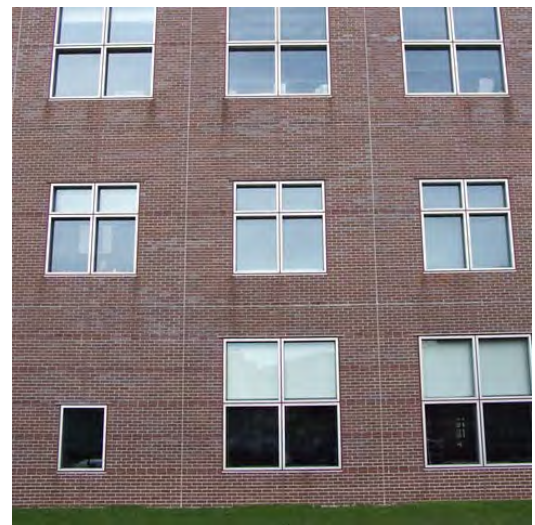
Figure 12: Placement of movement joints creates wall symmetry.
