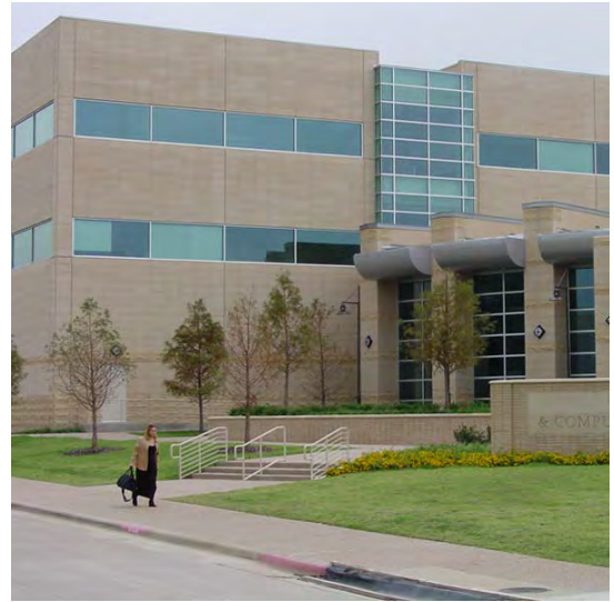
Figure 11: Movement joint integrated into design.
