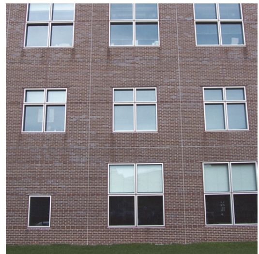
Figure 12: Placement of movement joints creates wall symmetry.
