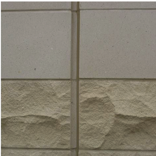
Figure 10: Movement joint placed at continuous notch in veneer.
