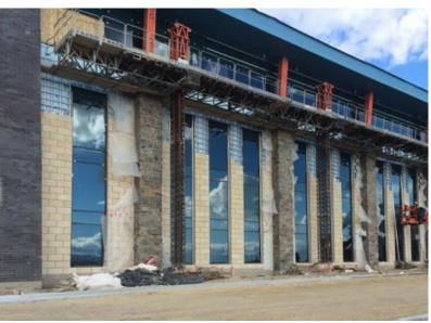
The ARRIS-clip thin stone was installed using the Gridworx aluminum stone hanging system and their Discrete Girt / Z-channel assembly, creating a back drained and ventilated open rainscreen façade and providing a system that provided the higher effective R-value they needed to achieve ASHRAE 90.1 compliance.
