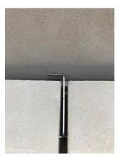
Now you can fasten anchor into the structural back up. Window sill units are now ready to be installed.
