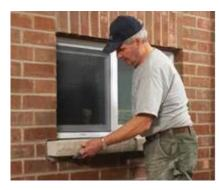
3. After final sill is in place, brush excess mortar from the surfaces utilizing uncoated steel and soft fibre brush.
