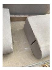
Site-cut slot openings into the bed of the window sill units to insert the tails on the split-tail anchor.
