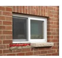
2. Insert Sill; repeat as required depending on window size (2 sills for this example.)
