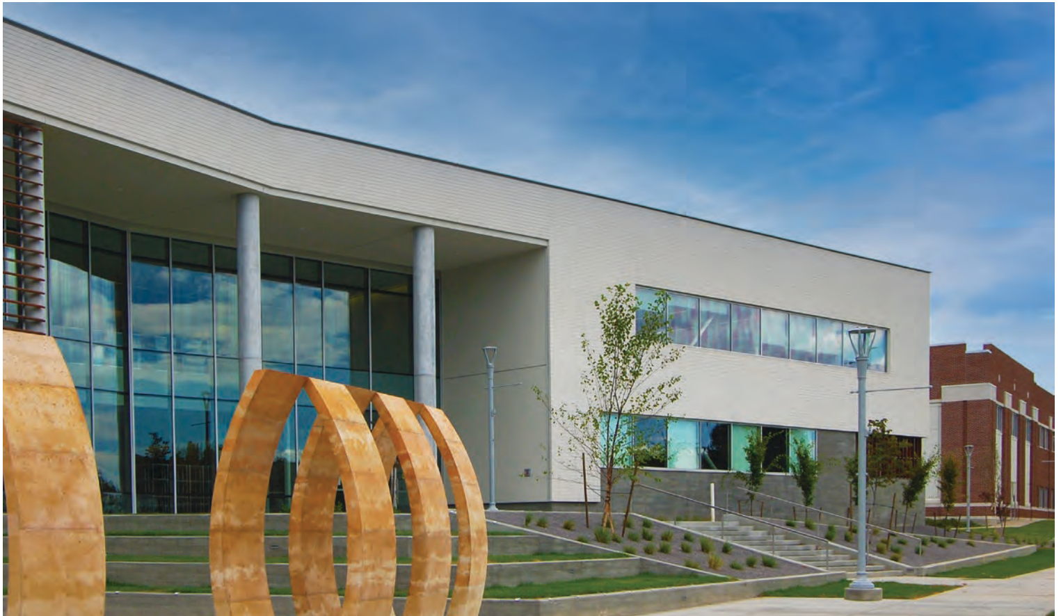
Arriscraft ARRIS-stack over ProGUARD DP® Insulated Cement Board Panels, using Laticrete MVIS materials.
