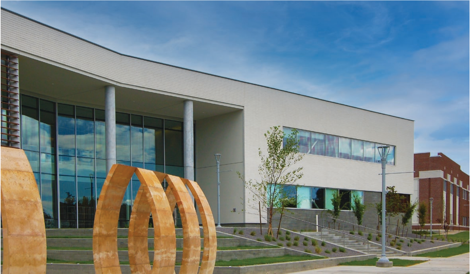
Arriscraft ARRIS-stack over ProGUARD DP® Insulated Cement Board Panels, using Laticrete MVIS materials.
