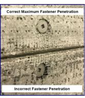
Ensure screw length selected allows for a minimum of 1" penetration into the concrete structural back-up. Calculation for minimum screw length:
