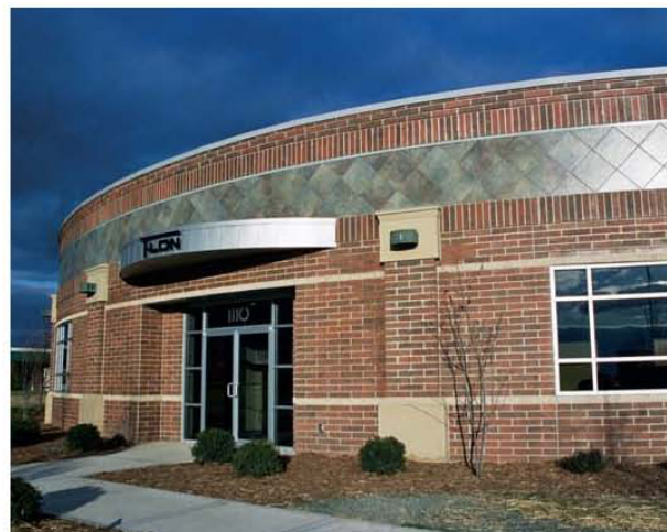
Single Wythe Half-High Construction in Hartland, Wisconsin
